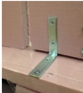
An L-bracket attached to the inner edge of the door frame.
