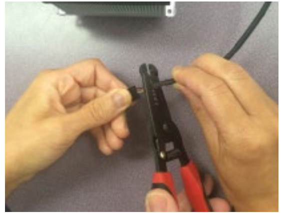
These teammates are working together to expose the colored wires and cut off the cap.
