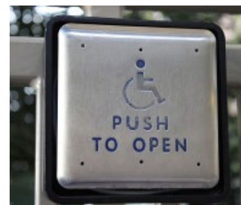
A push button activates a switch inside this door opener. Credit: Wikimedia Commons
