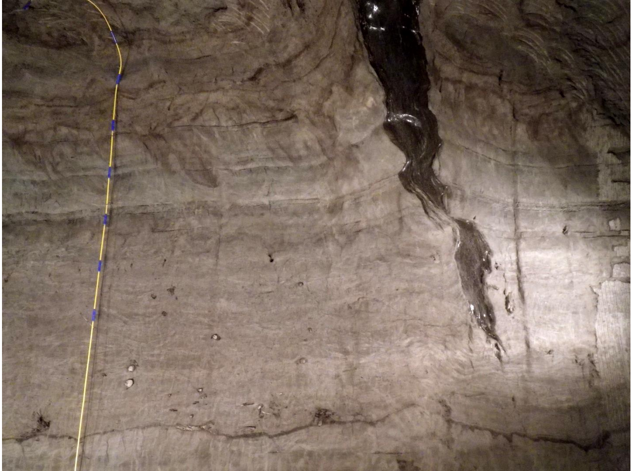
Figure S13. Small ice wedge in syngenetically frozen silt; note peat layers and numerous inclusions of organic matter. Left wall of the main adit of the new tunnel (T2), distance 23.0-27.0 m, elevation 229.2-231.5 m (for location, see Figure 6 ).
