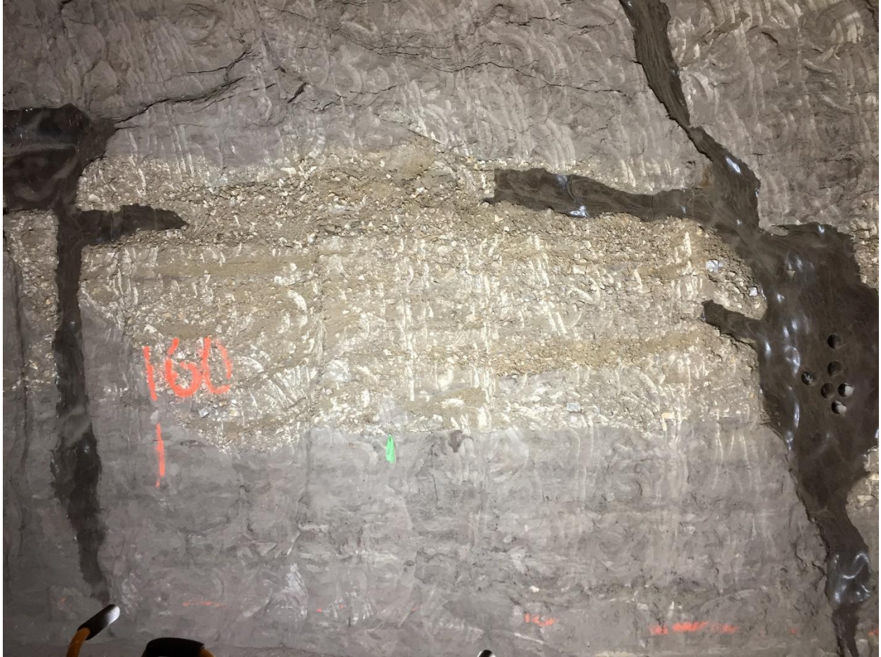
Figure S25. Layers of gravel and gravelly sand enclosed in Yedoma silt that were penetrated by 0.2- to 0.5-m-wide ice wedges. Layers of gravelly soils probably accumulated in thermo-erosional gullies. Note well-developed horizontal parts of ice wedges that are parallel to the gravel layers (for details, see Figure S26 ). Left wall of the main adit of the new tunnel (T2), distance 103.0-107.3 m, elevation 227.6-231.5 m (for location, see Figure 6 ).
