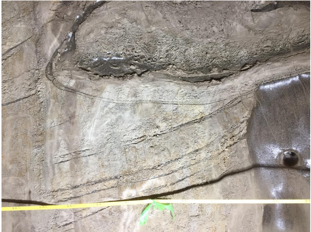
Figure S36. Syngenetically frozen Yedoma silt with ice belts and micro-cryostructures and syngenetic ice wedge affected by underground thermal erosion. Right wall of Crosscut #1 of the new tunnel (C1), distance 24.5-25.5 m, elevation 228.9-229.7 m (for location, see Figure 10 ).
