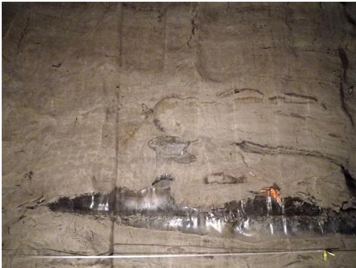
Figure S16. Large body of thermokarst-cave ice. Right wall of the main adit of the new tunnel (T2), distance 39.7-42.8 m, elevation 228.9-231.5 m (for location and interpretation, see Figures 6 and 7 ; for details, see Figures S17, S18, and S19 ).
