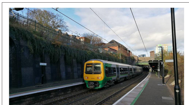
FIGURE 1 | Electric train and overhead contact wire on West Midland railway line, UK.
