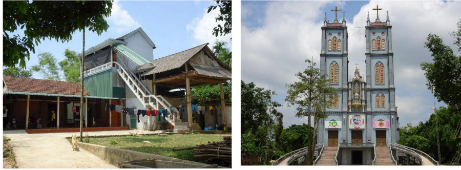
FIGURE 4 | Improved construction practice to cope with the potential floods.
