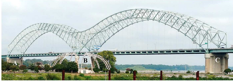
FIGURE 5 | Hernando Desoto (HD) bridge main spans (with Pier labels).
