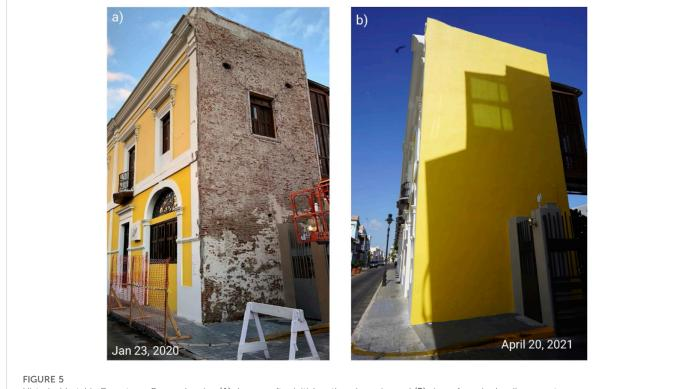
Historical hotel in Downtown Ponce showing (A) damage after initial earthquake series and (B) view of repaired wall segment.
