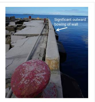
FIGURE 7 View of bowing of berth at Pier 2.
