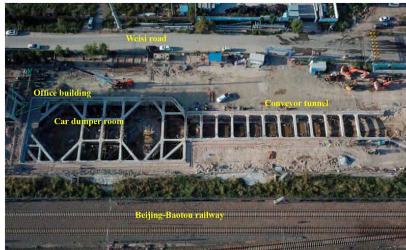
FIGURE 1 | Surrounding environment of the foundation pit.
