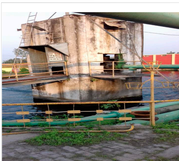
FIGURE 4 Fresh water reservoir.
