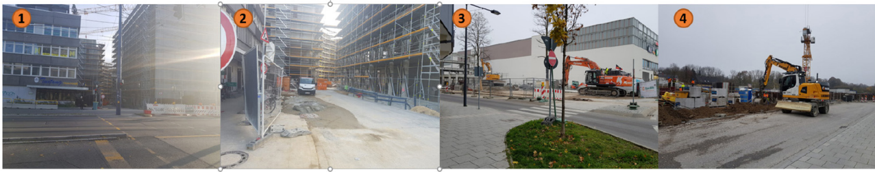
FIGURE 1 | (1) and (2) show the first, (3) and (4) the second investigated construction site.
