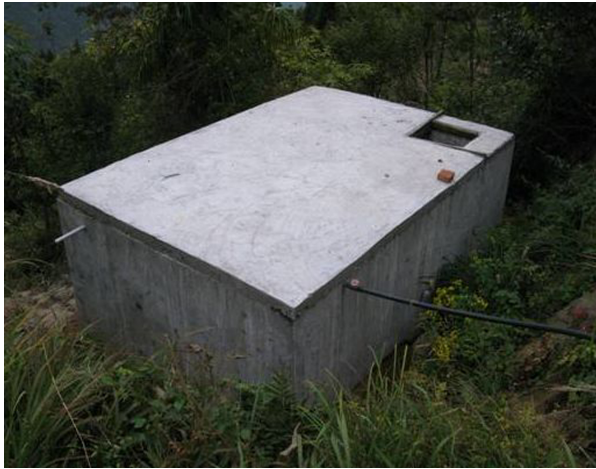
FIGURE 1 | The rural water reservoir commonly found in Guantao villages.
