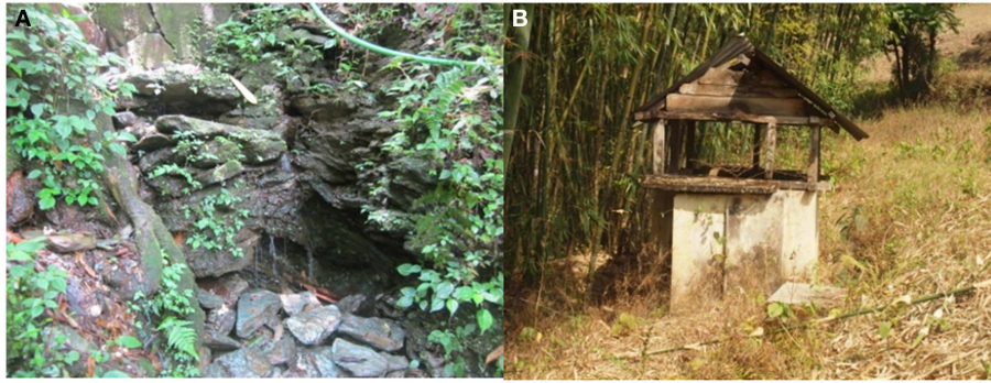
FIGURE 1 | Photograph of the study areas: (A) spring water (B) a typical community reservoir where water from the springs was stored before being distributed to the households.
