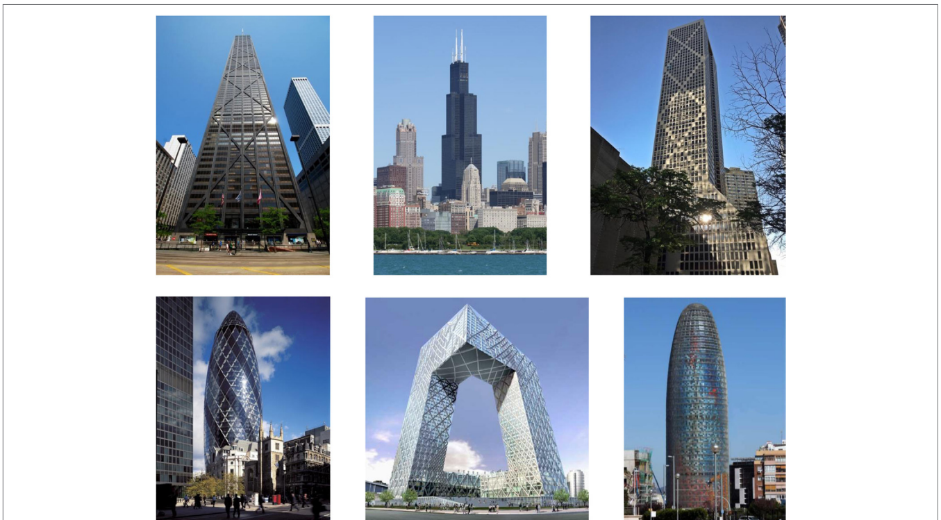
FIGURE 5 | From the top left, clockwise: John Hancock Building (courtesy of Royce Douglas); Sears Tower (courtesy of Michiel Van Dijk); Onterie Center (courtesy of Marshall Gerometta); Agbar Tower, Barcelona (courtesy of Mary Ann Sullivan); CCTV, Beijing (courtesy of Office for Metropolitan Architecture); and 30 St. Mary’s Axe, London (courtesy of Nigel Young).
