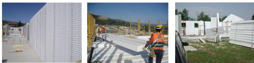
FIGURE 9 | Examples of installation of formwork in site (courtesy of Nidyon Costruzioni).
