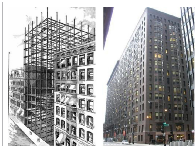
FIGURE 2 | From the left: Unity Building, Chicago (courtesy of Chicago History Museum); Monadnock Building, Chicago (courtesy of David K. Staub).
