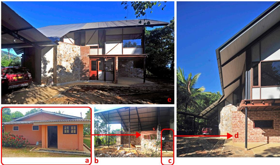
**FIGURE 10** Mountain house. (A) The old house on site; (B) the new structure and roof ‘sheltering’ the retained fabric; (C) kabok bricks ‘found’ on site; (D) the new, reused kabok brick wall defining the entrance to the house; (E) the bricolage-like formal language accommodates a seemingly-random mix of new and ‘found’ material: stone, clay bricks, kabok bricks, timber, lath and plaster, steel structural skeleton, metal roofing, etc.
