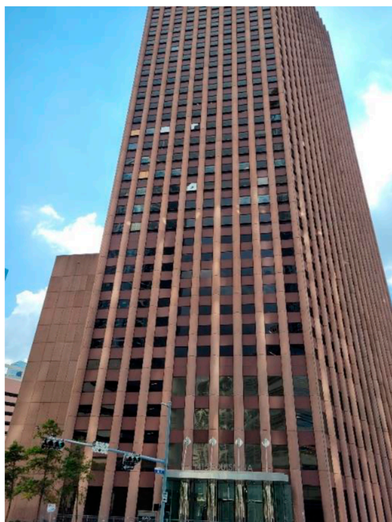
FIGURE 12 Damage sustained by the wedge international tower during hurricane Beryl (Kalliontzis et al., 2024).
