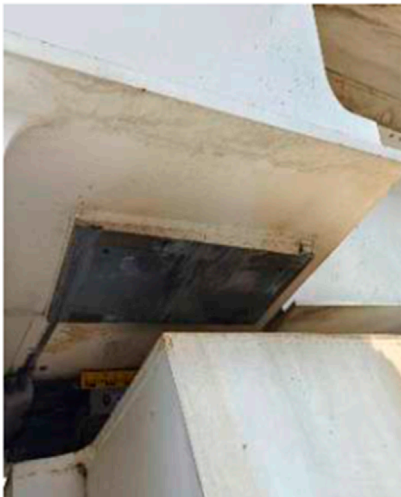
Pot bearing damage
