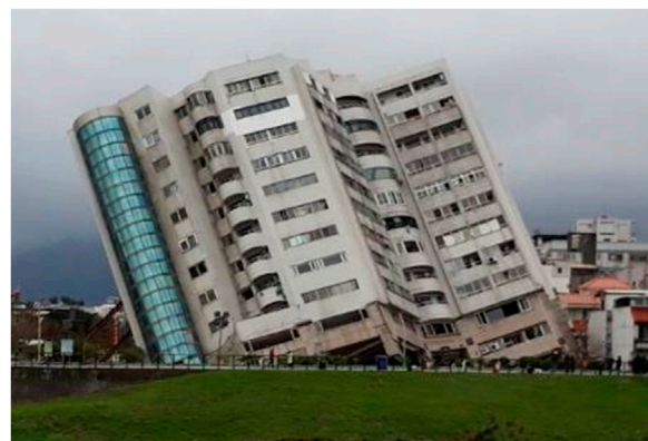
FIGURE 11 Severely tilted soft and weak story building (Yun Men Tsui Ti Building) in the 2018 Hualien earthquake.
