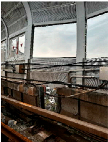
Sound barrier deformation and damage
