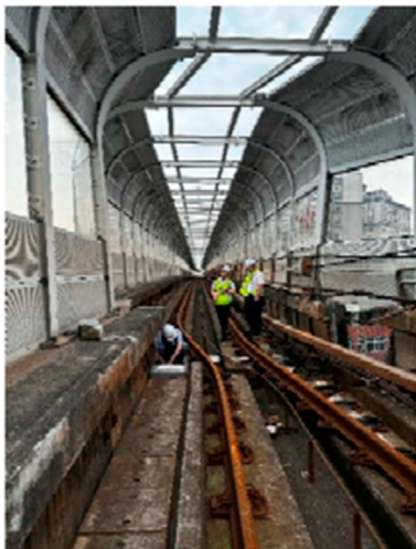
Track displacement and deformation
