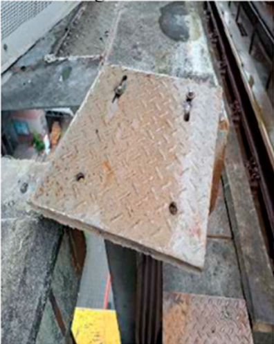
Bridge parapet displacement and damage
