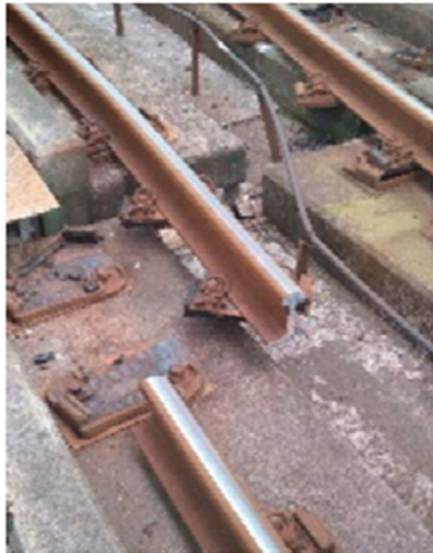
Steel rail deformation and fracture
