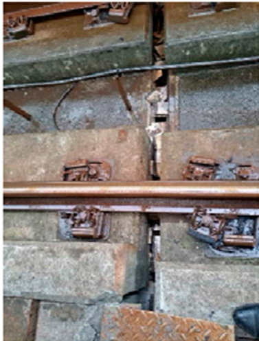
Base plate failure/damage
