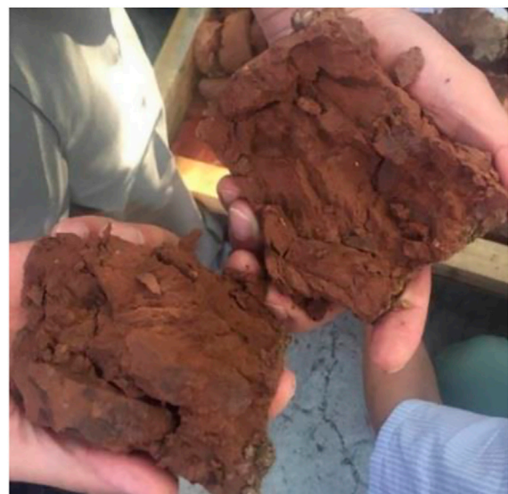
FIGURE 11 Mudstone at the pile tip in Project Example 1.
