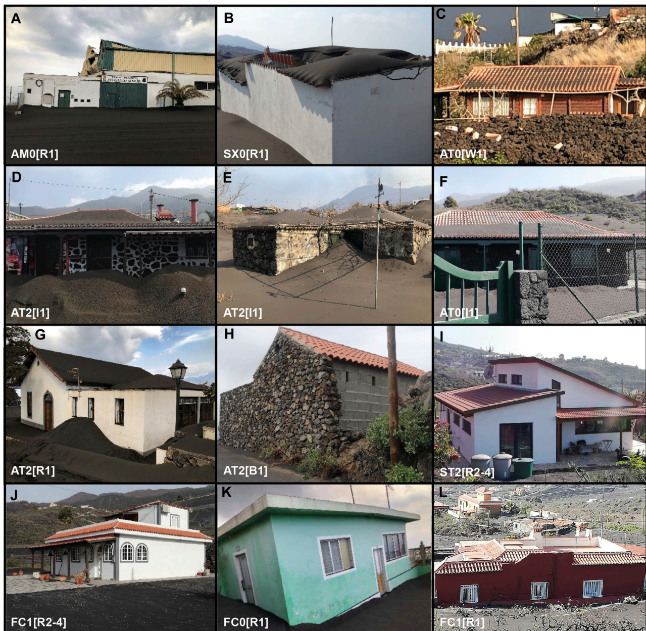
FIGURE 3 Roof and building types identified in our survey. Examples of Weak, WE (A–C); Medium Weak, MW (D–F); Medium Strong, MS (G–I); and Strong, ST (J–L) classes are displayed.
