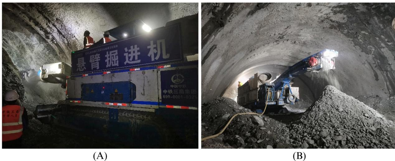
**FIGURE 9** Photographs of upper benching cantilever road header construction: (A) excavation of upper benching and (B) rapid slag discharge.
