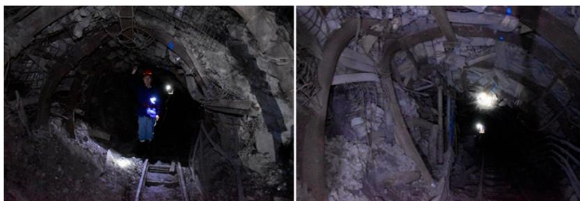
**FIGURE 1** Deformation of surrounding rock of roadway buried -600 m in Xin'an Coal Mine. (The support components on the right side undergo characteristic failure due to the action of stress).
