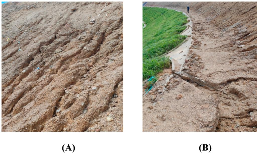
FIGURE 4 Slope erosion damage (A) Rill and shallow gully erosion (B) gully erosion.
