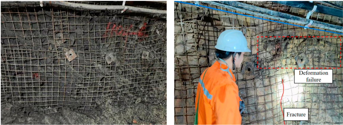
FIGURE 1 Schematic diagram of roadway deformation and support methods.
