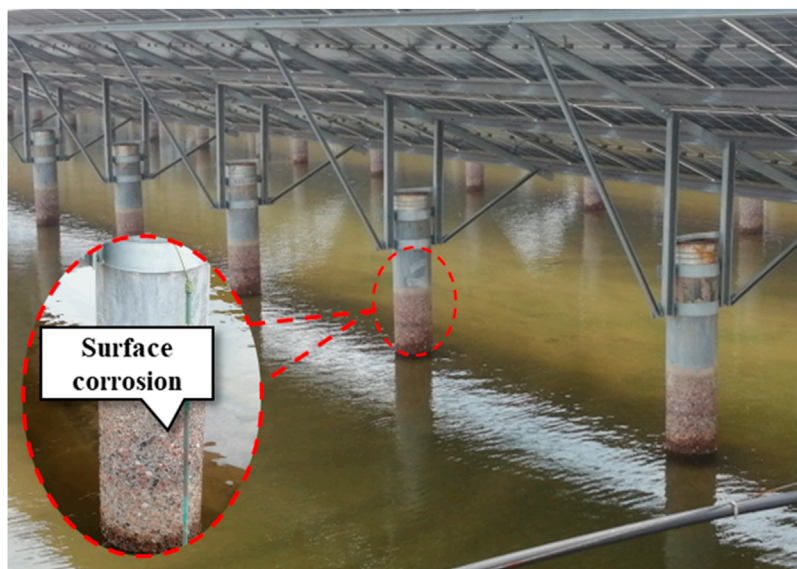
FIGURE 1 Corrosion condition of photovoltaic PHC pipe pile foundations.
