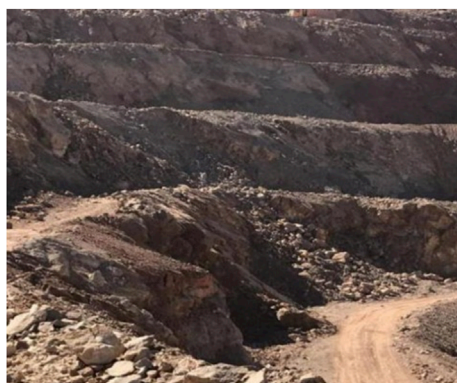
FIGURE 3 Multi-step landslides and platform cracks on mine slopes.
