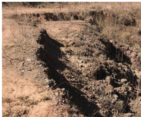
FIGURE 2 Minor landslides on mine slope terraces.
