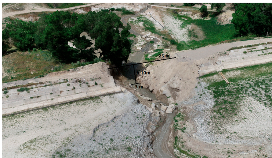
FIGURE 6 3D model of the Voroshilov reservoir dam breach, obtained by lidar surveying.
