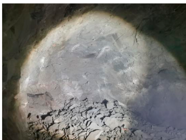
FIGURE 6 Blasting effect of the proposed test scheme.
