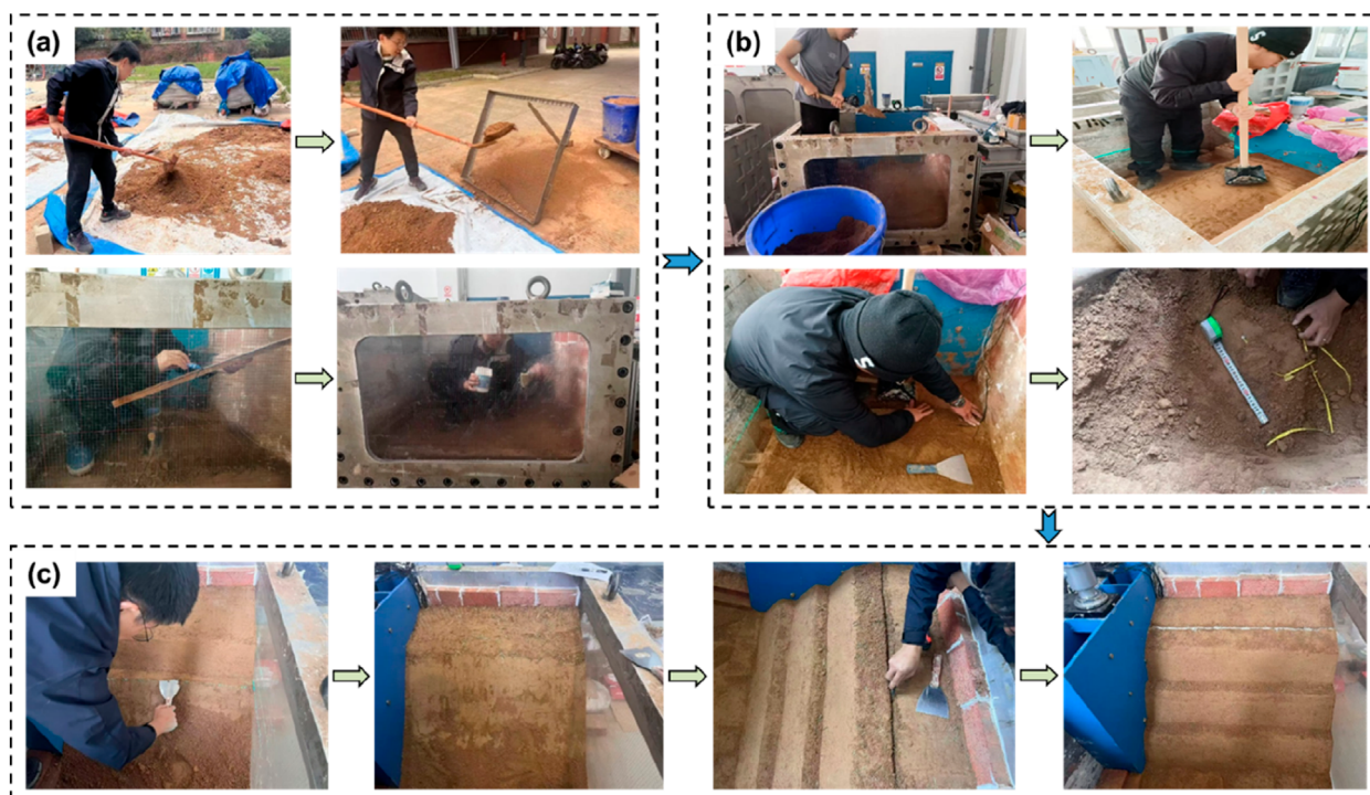
FIGURE 6 Construction process of the terraced loess slope model: (a) Preparation of soil and model box, (b) Filling soil and sensor arrangement, and (c) Slope excavation and crack construction.
