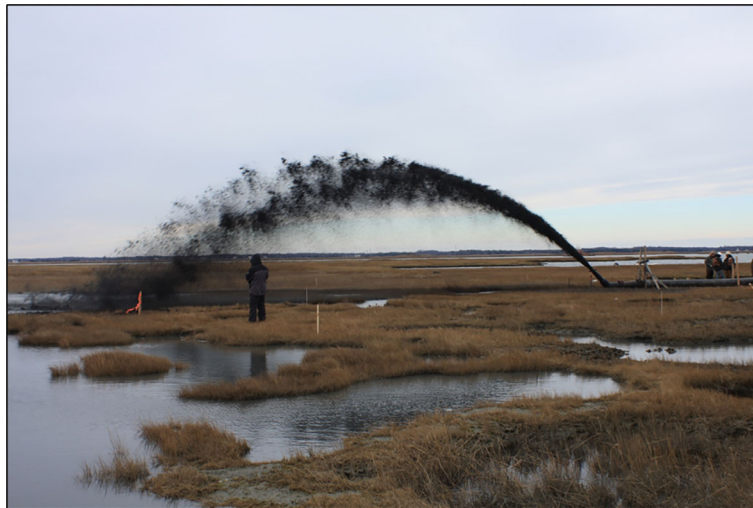
FIGURE 2 High-pressure slurry marsh amendment technique for thin-layer placement (TLP) in the Avalon, New Jersey, USA. marsh (source: USACE).
