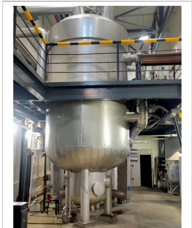
FIGURE 1 | Vessel of the COSTTHES facility.
