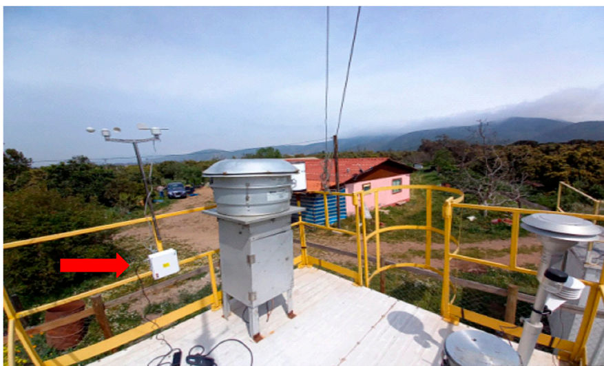
FIGURE 3 | Low cost monitoring station in Los Caleos (arrow). To the right is the sample inlet for the BAM-1020 monitor.
