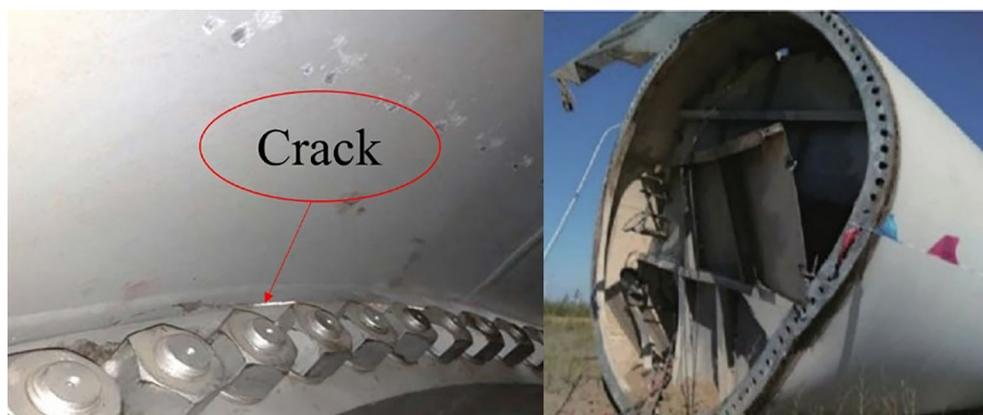
FIGURE 2 Fatigue cracks and fatigue failures of inland wind turbine towers (Zou et al., 2021).
