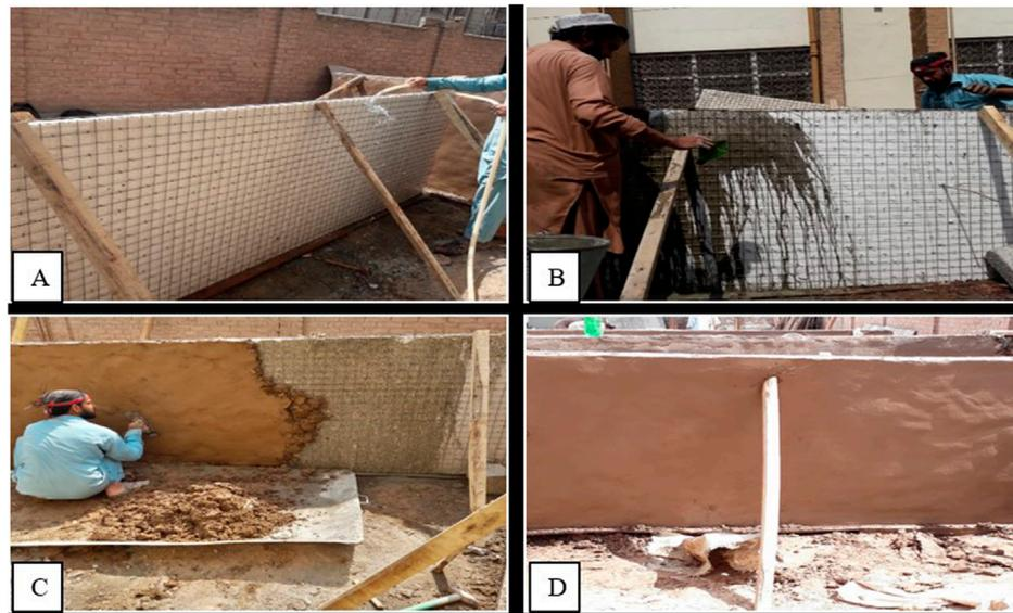
FIGURE 2 Casting of SMIP's (A) sprinkling water (B) application of grout (C) stabilized mud plastering (D) finished surface with trowel.
