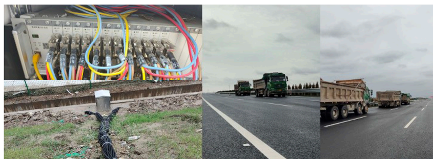
FIGURE 3 Pavement structures monitoring system and field loading test.
