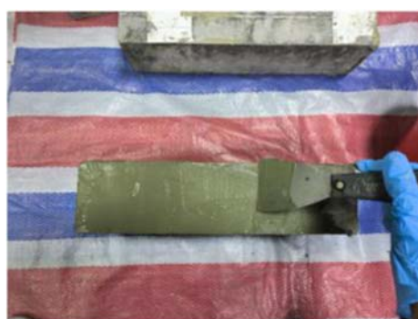
Application of cementitious osmotic crystalline coating
