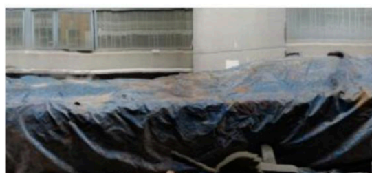
4. Steam curing of prefabricated beams
