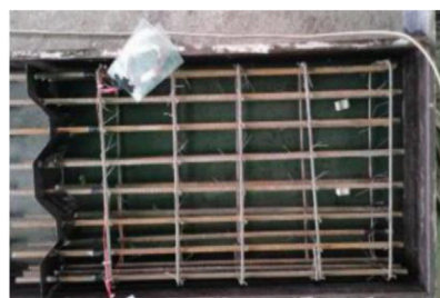
1. Reinforcement and formwork
