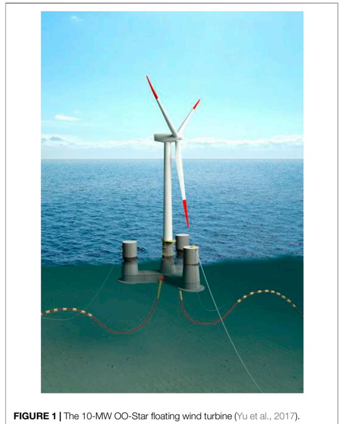
**FIGURE 1** | The 10-MW OO-Star floating wind turbine (Yu et al., 2017).
