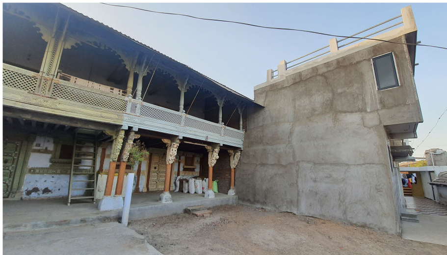
FIGURE 8 Image showing hybridisation of the façade 1 (Source: Photograph by Author, May 2023).
