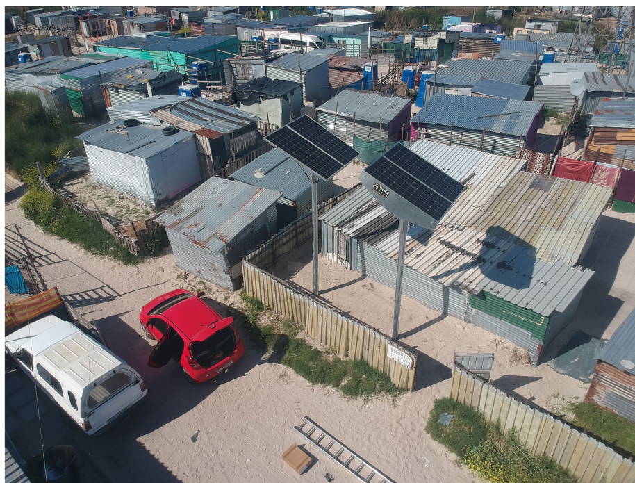
FIGURE 3 Solar microgrids being installed in Qandu Qandu, Cape Town.
