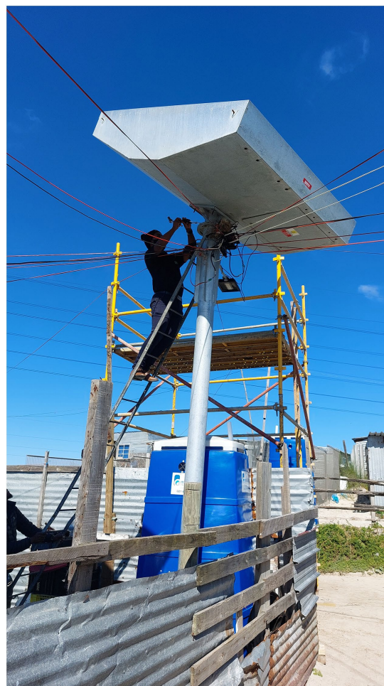
FIGURE 2 Installing a solar tower-based microgrid in Qandu Qandu, Cape Town, 2021.
