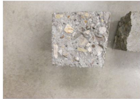
FIGURE 9 | Unlined (control) beam after to flexural testing.
