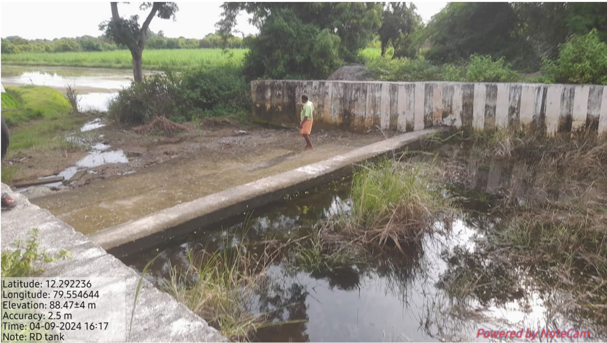
FIGURE 4 Leaking surplus weir.
