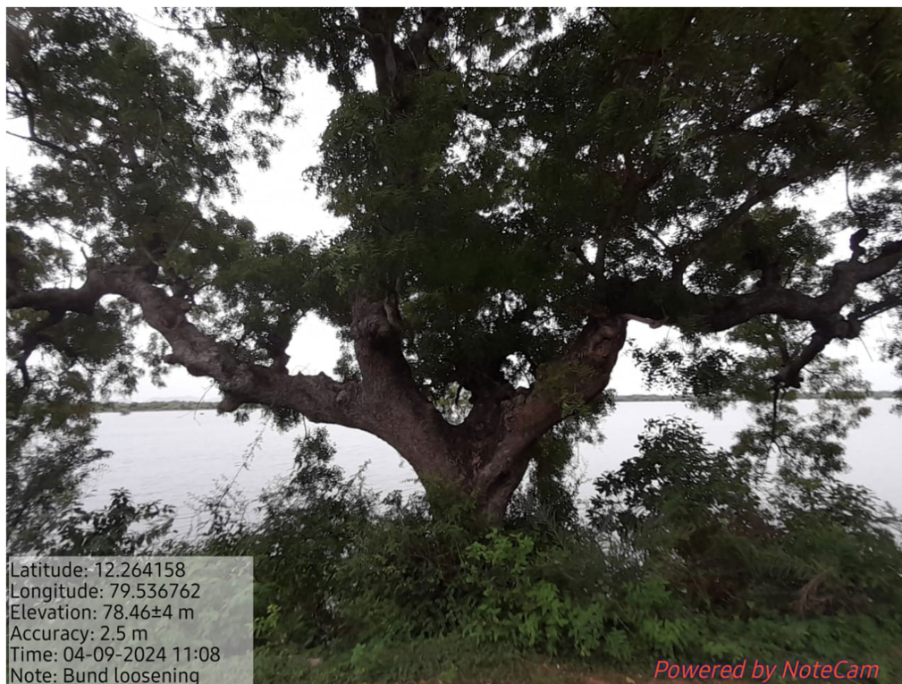
FIGURE 9 Growth of a Huge tree—weakening the tank bund.
