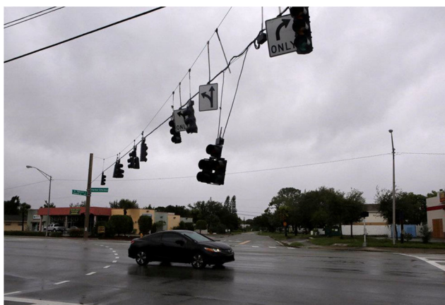
FIGURE 2 | Typical span-wire traffic signal system.
