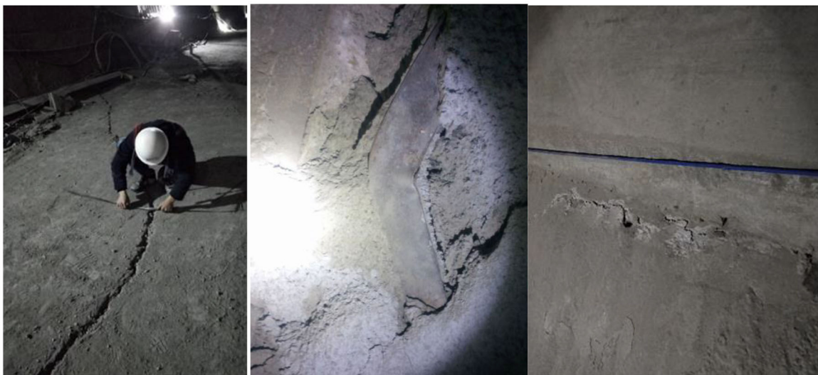
FIGURE 2 | Deformation of major tunnel lining.
