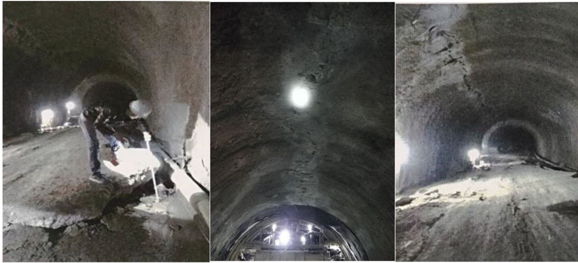
FIGURE 1 | Initial support failure.
