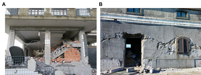
FIGURE 1 | (A) Damage to reinforced concrete building at Mazzasette ( I = 8 EMS) and (B) to masonry edifice at Testa di Viperà ( I = 7-8 EMS).
