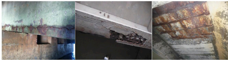
FIGURE 1 | Typical durability damage of harbor structures induced by chlorides.
