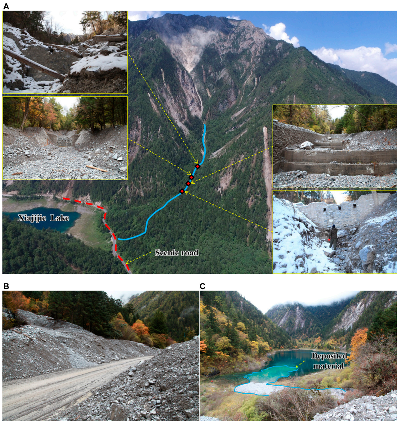
FIGURE 3 | View of Xiajijie Lake Gully. (A) Control engineering layout of Xiajijie Lake Gully (before the debris flow event on June 21, 2019). The blue line in the figure represents the main channel; (B) Debris flow material deposited on the scenic road on September 25, 2017; (C) Debris flow material entering Xiajijie Lake on September 25, 2017.
