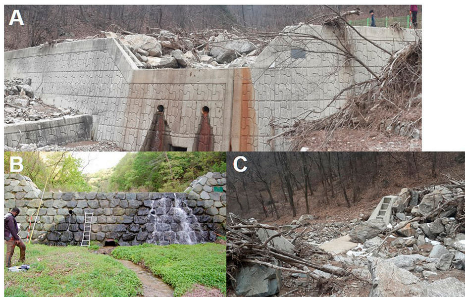
FIGURE 2 | Front views of (A) concrete, (B) stone check dams, and (C) The debris and driftwood laden check dam. The check dams in figures (2a) and (2c) effectively captured the rivers' debris and driftwood.
