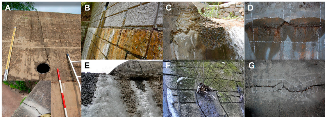
FIGURE 7 | Various deterioration types observed on concrete check dams. (A) vertical through crack and displacement caused by drying shrinkage cracking; (B) water leakage from a gap in a horizontal construction joint; (C) exposed aggregate and spalling, respectively, due to erosion at the spillway; (D) leakage and efflorescence at a horizontal construction joint; scaling and spalling of the downstream face due to freezing and thawing; (E) (F) uncontrolled vegetation around a drainage channel; (G) through crack and dam crest stepping.
