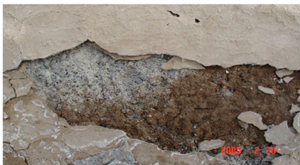
FIGURE 4 | Thaumasite formation under external sulfate attack (groundwater [\text{SO}_4^{2-}] = 653 \text{ mg/L} ) in the Yongan Dan in Keshi of China (Mingyu et al., 2006).
