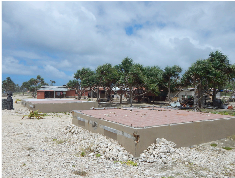
FIGURE 1 | Only the foundations remain from this beachfront resort on Efate Island after Cyclone Pam struck the area. Source: Author's own.
