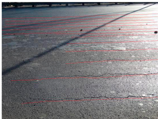
FIGURE 2 Longitudinal cracking on the asphalt pavement.
