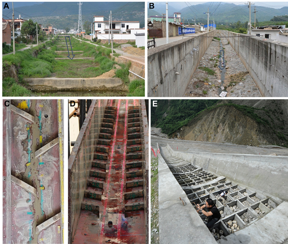
FIGURE 1 | Different types of debris flow drainage channels (A) Dongchuan-type; (B) V-type; (C) SIS-type; (D) OSS-type; (E) PRCB-type.
