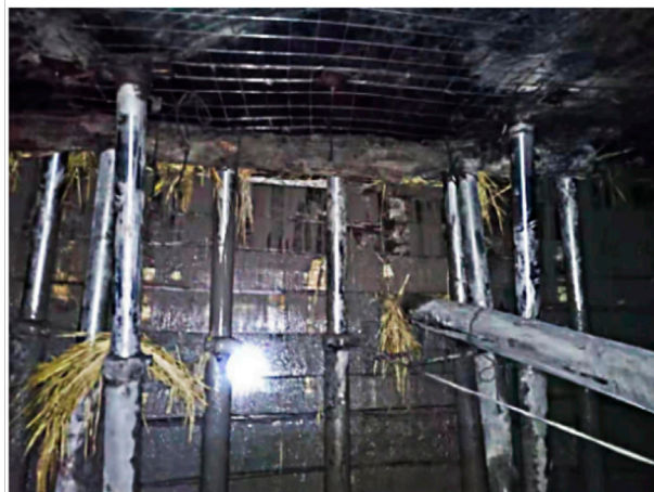
FIGURE 7 Design and construction of a paste baffle.
