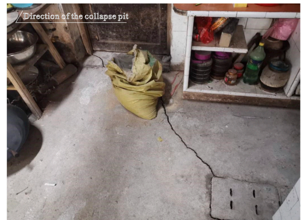
FIGURE 3 Tensile cracks in house No. 3.
